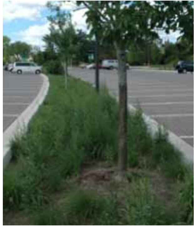
Vegetated swale in parking lot
