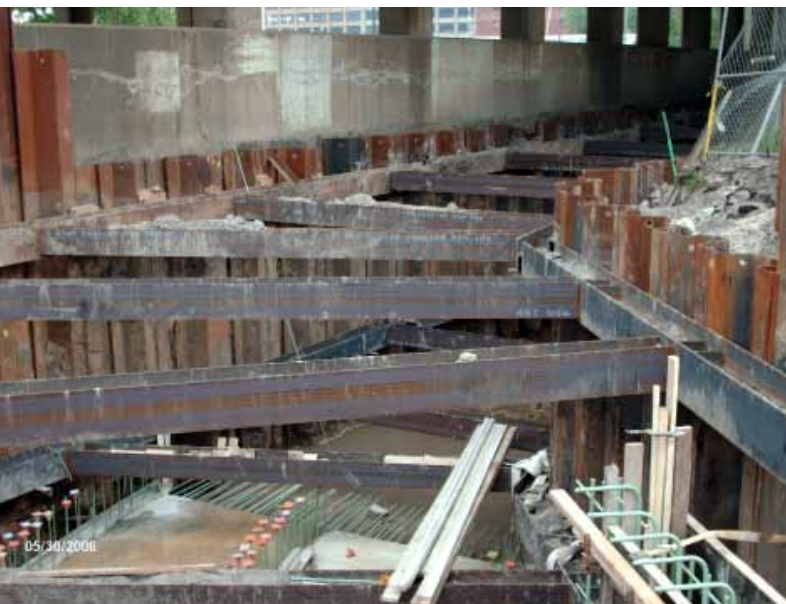
Combined sewer separation project in Grand Rapids
