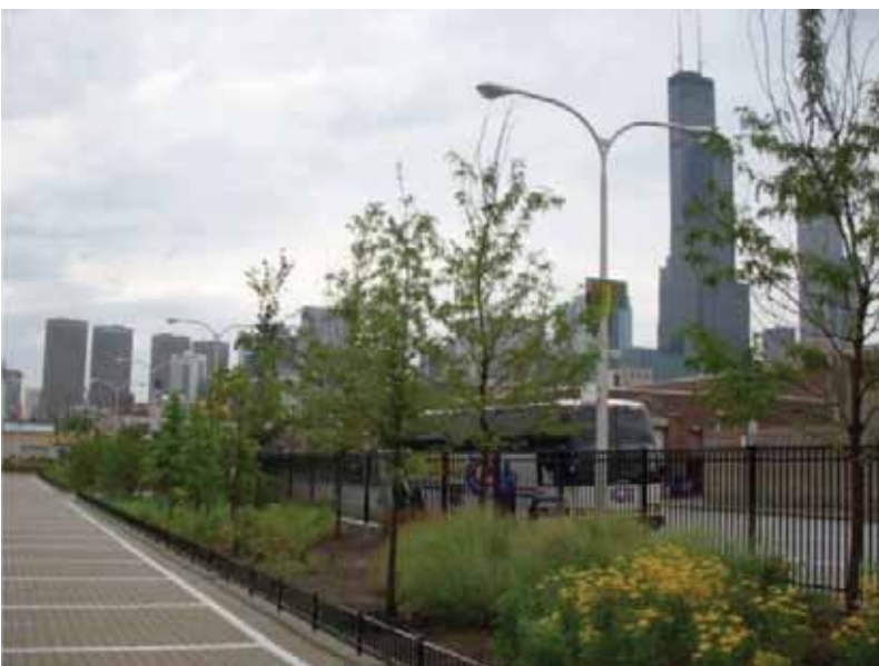
Porous pavement at Maxwell Street Market in Chicago
