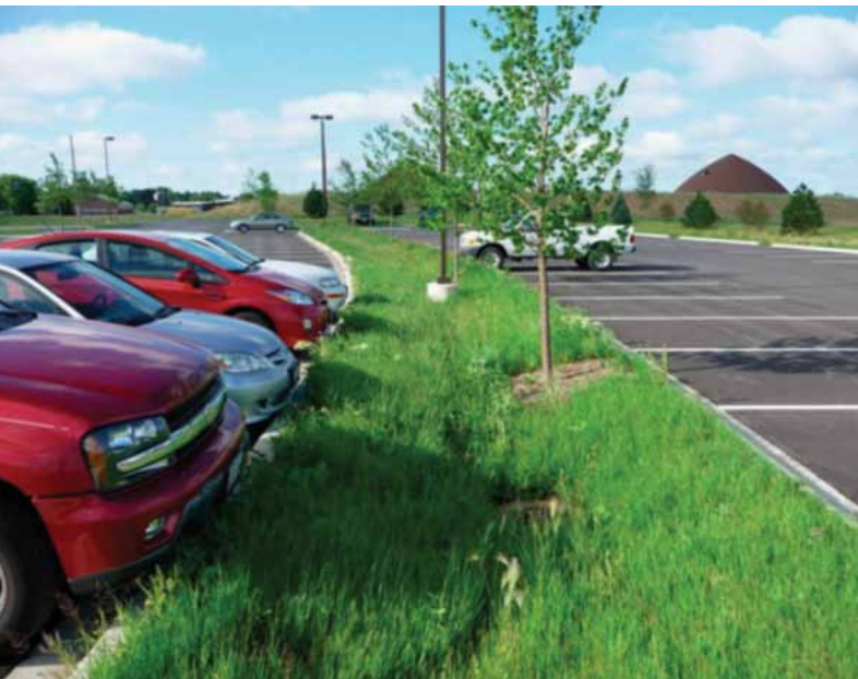
Vegetated swale in a parking lot
