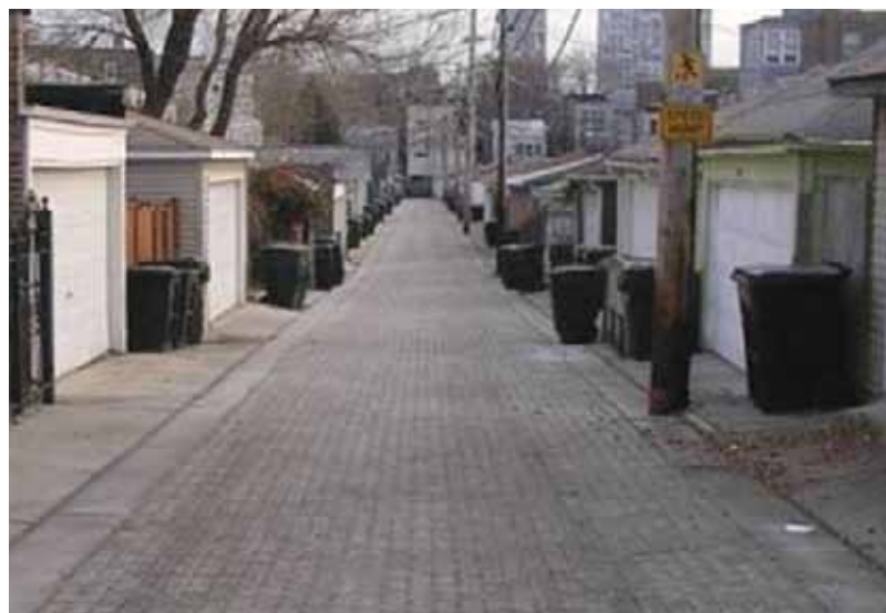
Porous pavement in an alley
