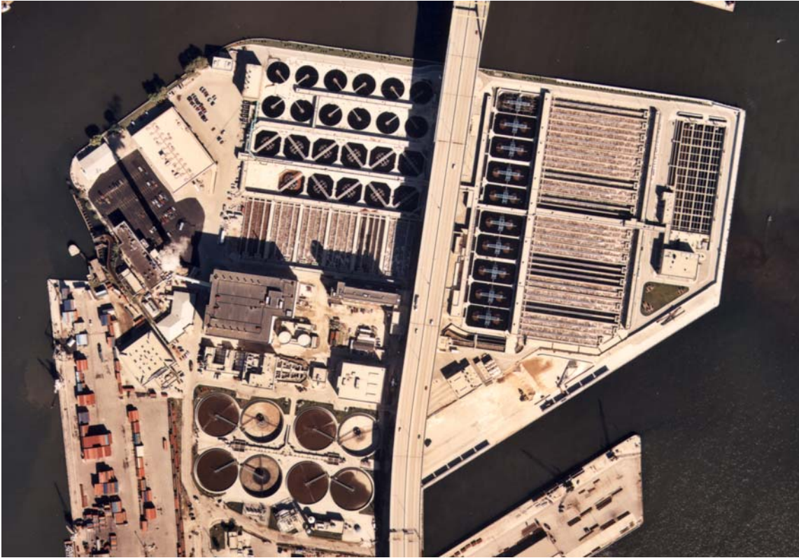
MMSD's Jones Island Water Reclamation Facility
