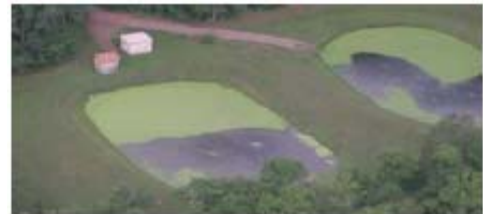
Previous WWTPs in the City of Bayfield (top photo) and Pikes Bay Sanitary District (lower photo)
