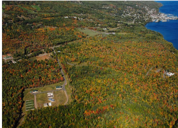
New Greater Bayfield Wastewater Treatment Plant which Serves the greater Bayfield region and provides a zero percent effluent discharge into Lake Superior.
