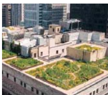
Green roof on top of Chicago's City Hall.
